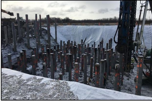
Figure 2: Large group of driven PPCH piles
