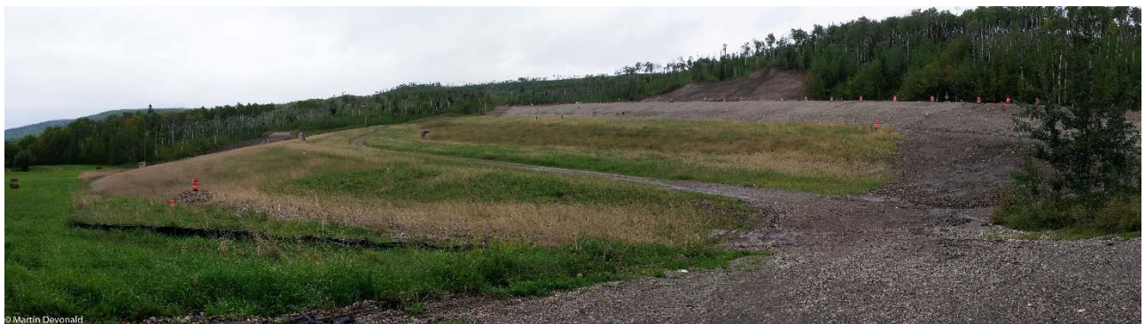
Figure 7. New "Military Berm" fill embankment in 2016; one-year post construction.
