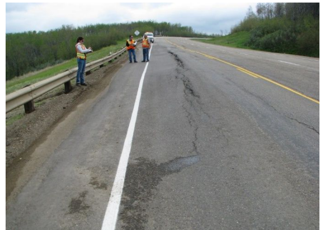
Figure 1. Drop in the pavement on the east-bound lane of the embankment on Highway 986:01 in June 2012
