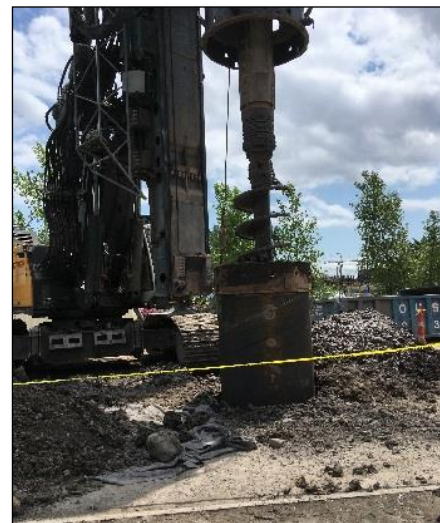
Figure 2. Casing placement and soil excavation
