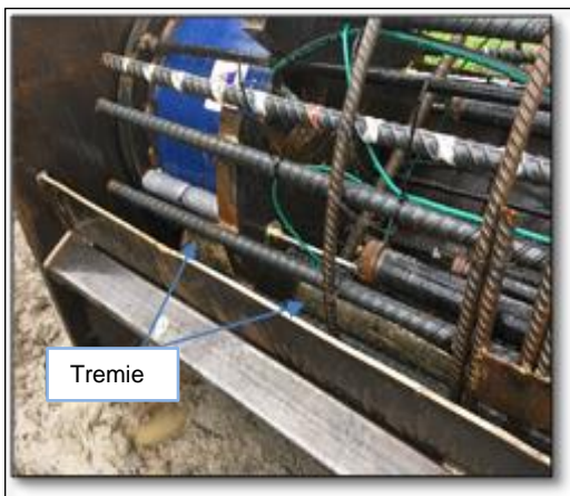
Figure 3. Rebar cage & load tests assembly
