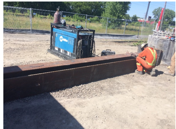
Figure 4. Lateral Load Test Setup
