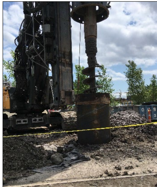
Figure 2. casing placement and soil excavation
