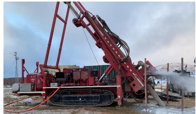
Figure 8: Drilling of backfill hole (12-inch) at stope M-1A
