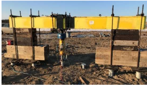
Figure 3. Pile load test setup
