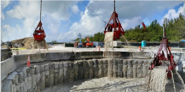
Figure 6. Excavation of the secant pile launch shaft “in the wet”
