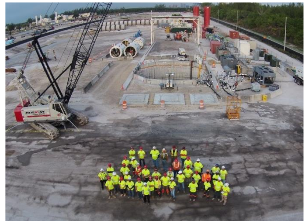
Figure 7. The construction team
