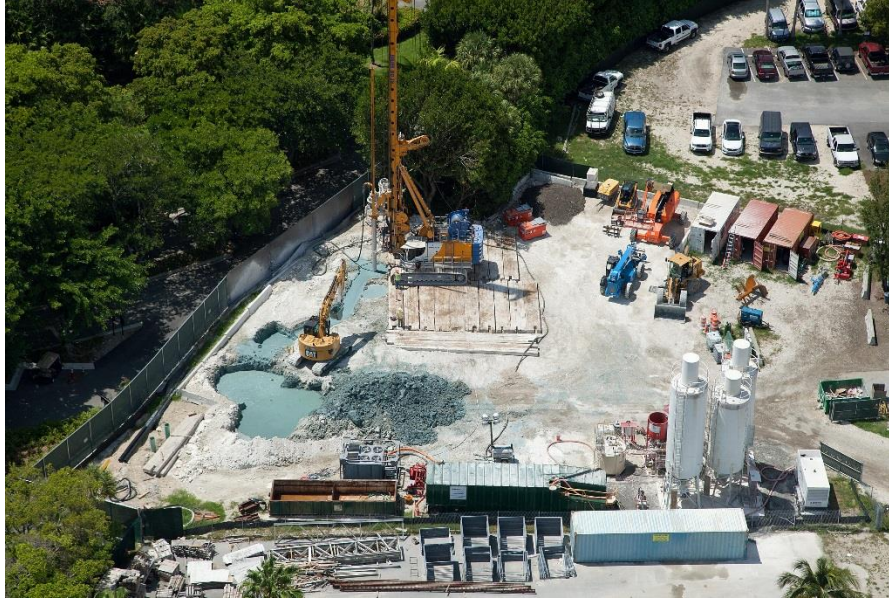
Figure 8. Deep Soil Mixing on Fisher Island
