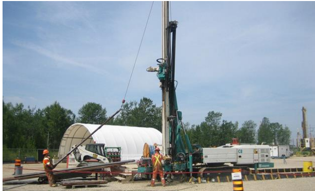
Figure 7 The equipment used for drilling
