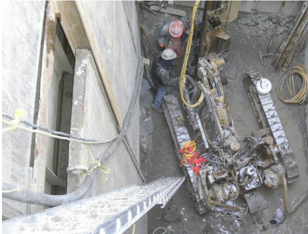
Figure 5 Compaction grouting in progress inside a shored excavation
