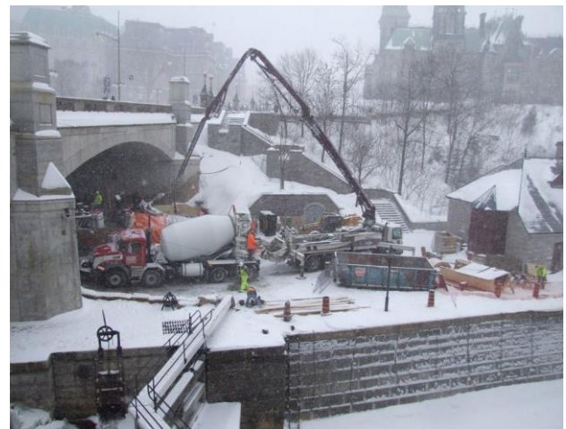
Figure 9 Permeation grouting at Rideau Regulator Chamber
