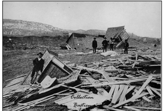
Figure 9. Destroyed houses due to a landslide and displacement wave (April 1908) in Notre-Dame-de-la-Salette, QC, located roughly 40 km north of Ottawa (Photo: GSC Library).
