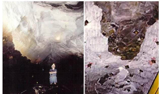
Figure 19: Slabbing in the competent sandstone layers due to high horizontal stresses in eastern Sydney (after Oliveira and Diederichs 2017).
