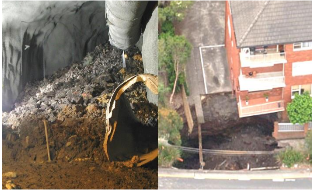
Figure 13: Collapse and chimney failure due partially to upward weakening beds and Voussoir beam surcharge
