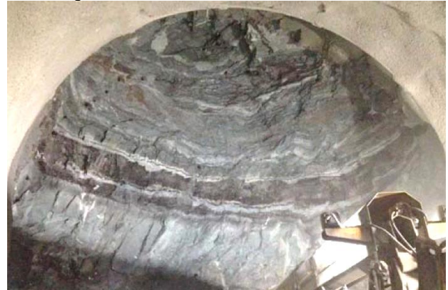
Figure 11: Roof instability due to thinning beds
