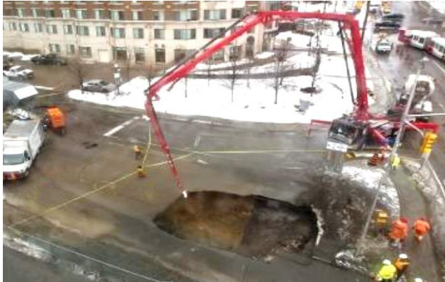
Figure 14: Roof collapse above subway construction due to weak rock/soil surcharge above thin roof beam
