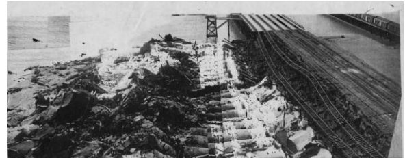
Figure 6. The United Grain Growers Limited Current River Terminal After Failure. (Courtesy: Viterra Inc.)
