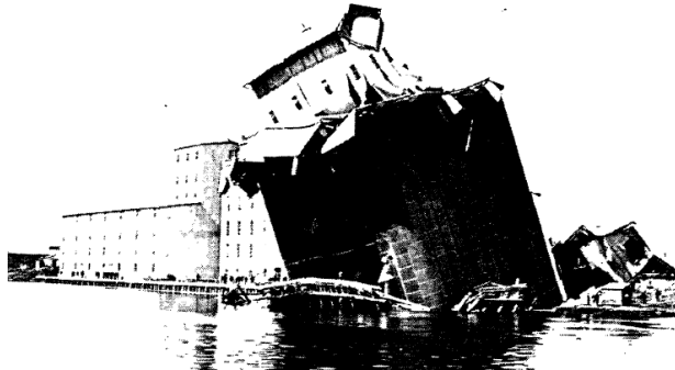
Figure 5. Ogilvie Elevator in its Failed Position (Courtesy: The Thunder Bay Museum)
