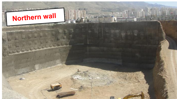
Figure 2. Longitudinal profile of the excavated northern wall [Poormousavian and Fagher 2017]
