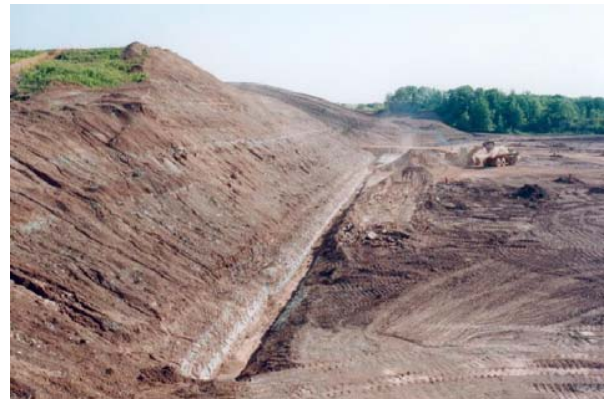
Figure 9. A cutting trench to release horizontal high ground stress
