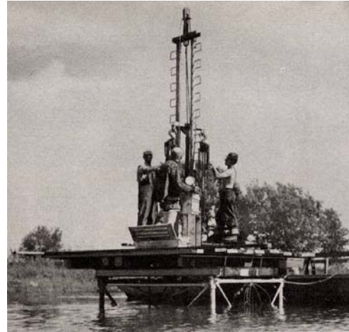
Figure 2. Drill crew operating Swedish Foil Sampler
