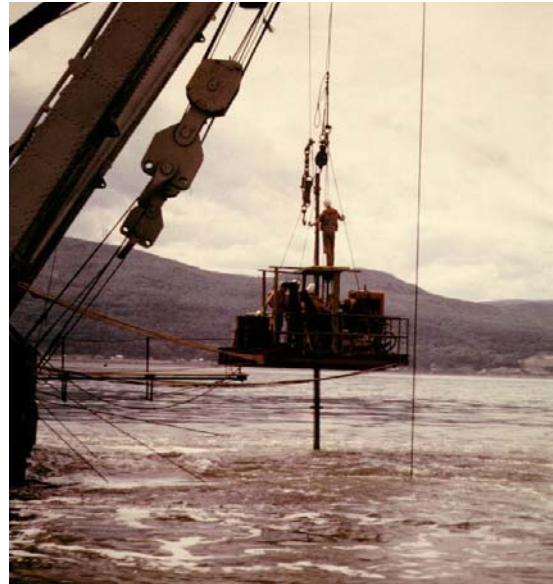
Figure. 6 Drillers working from the Stationary Cable Rig
