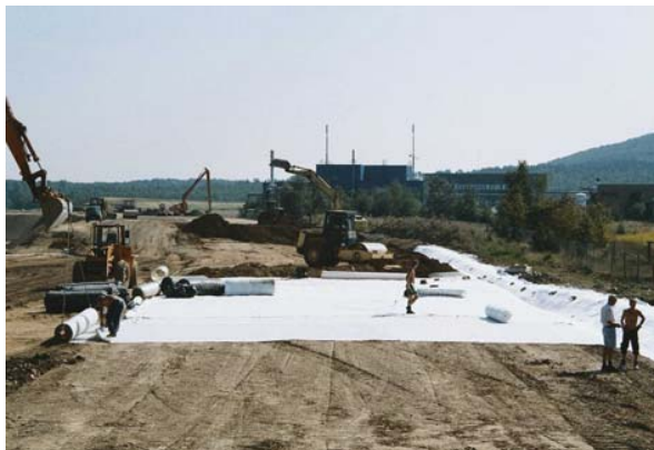
Figure 5. Installation of geosynthetics in the infrastructure sealing application by-pass road B 82n Langelshiem, Germany
