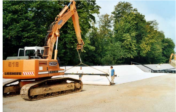
Figure 4. Installation of the needle-punched geosynthetic clay liner serving as RiStWag sealing in the project B 3 Wasser near Freiburg
