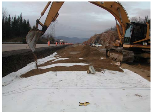
Figure 7. Cover soil placement of the GCL seams. Technique used to prevent the movement of the membrane and the seams during the soil placement operations by Bulldozers as shown in Figure 3.
