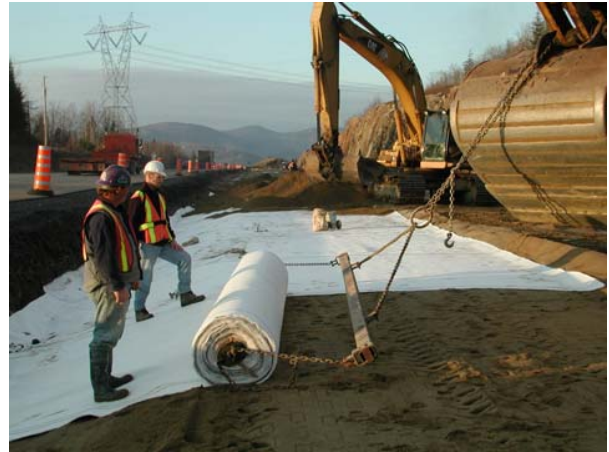
Figure 6. Deployment of the GCL for the future Autoroute 73/existing Route 175 in Stoneham, Quebec.
