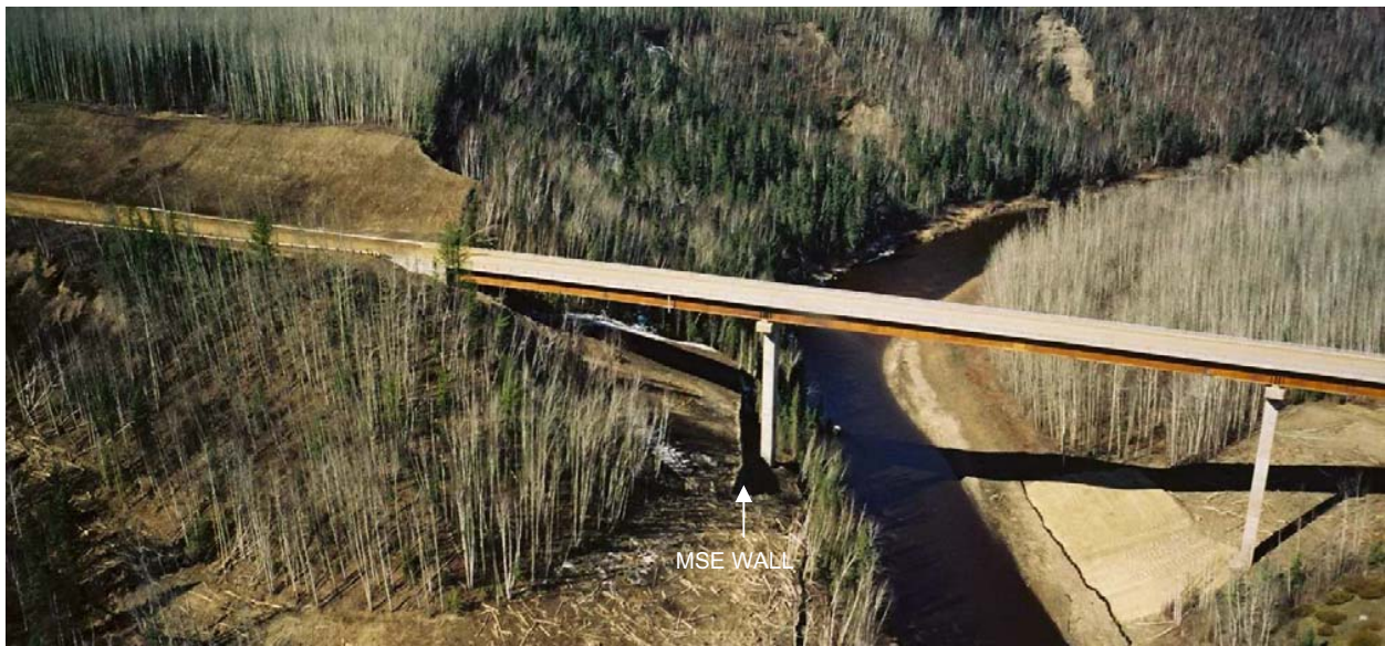
Figure 6. Photo of the Completed Bridge and Shear Key / MSE Wall Looking Southwest
