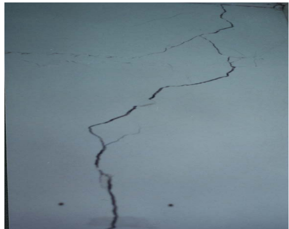
Figure 4. Fissures inside the Armenian School.
