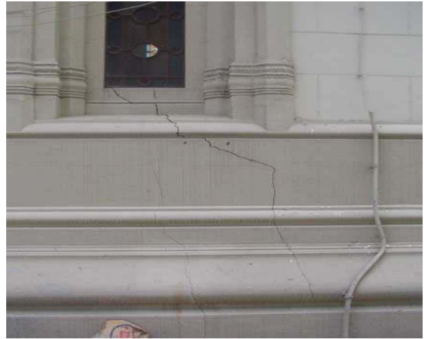
Figure 3. Fissures along Armenian Church wall.
