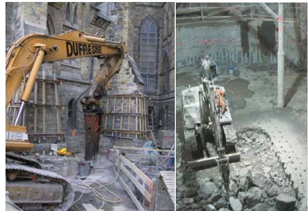
Figure 5: 66 kW Hoe Ram as used to excavate the upper portion of the Access Shaft (left). 25 kW Hoe Ram working in the Mechanical Room (right).
