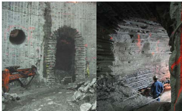
Figure 8: Final excavation profiles showing tight line drilling and good wall control for the Mechanical Room wall, Stair 'B' Tunnel (left) and LOP Tunnel (right).
