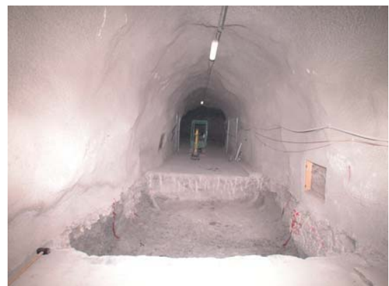
Figure 4. View of the northern entrance gallery after removing the reinforced concrete slab
