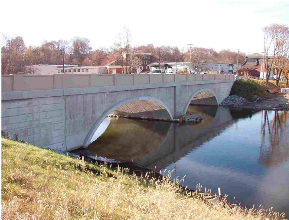
Figure 8. Completed TechSpan Arch structure on Pile Foundation Jamestown, New York
