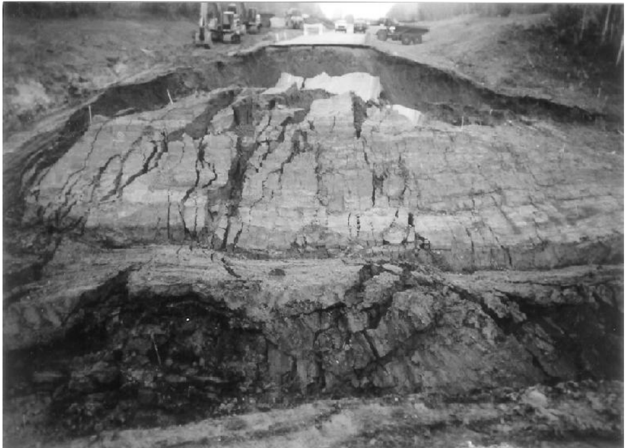
Figure 2: Excavation Slope Failure, Hwy 88 Culvert Replacement Project
