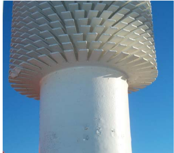
Figure 2. Close-up photo of the radiator of the thermosyphon installed at the Giant Mine.
