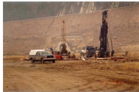
Figure 4. Geotechnical investigations at the downstream toe of the dam
