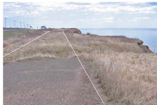
Figure 6. Road setback, Route 132, Bonaventure, QC, showing former highway in foreground (marked by white lines), truncated by gullies intersecting the coastal cliff at right, and present highway (beside power poles), set back further from the coast at left (DLF, Geological Survey of Canada, 2004-05-09).
