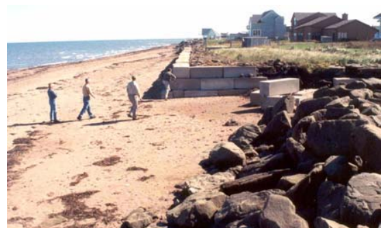
Figure 7. Increasingly large and expensive homes are being built on ocean-front land in many areas. This shows a variety of shore-protection structures at Barachois, NB, where the sand supply is very limited and rapid coastal retreat is the norm (DLF, Geological Survey of Canada, 2002-09). This was also one of the areas badly hit by sea-ice pile-up onshore in January 2000, when ice penetrated into the interior of some homes.
