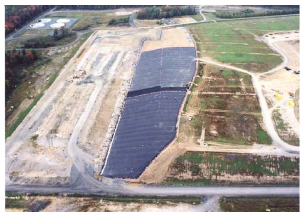
Figure 7. Quebec's first MSW piggyback installation.
