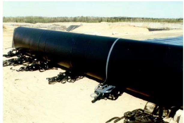
Figure 8. Prefabricated polyethylene geomembrane rolls with plastic spacers.
