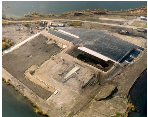
Figure 6. Contaminated soil cap closure.
