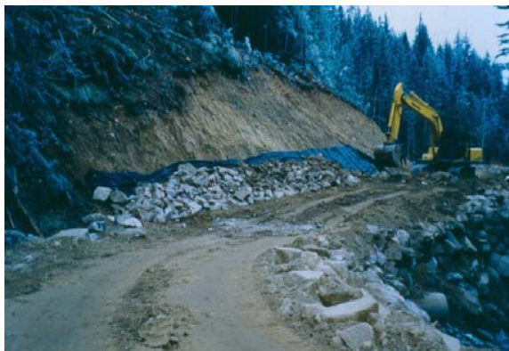
Figure 2. Unrolling the geotextile
