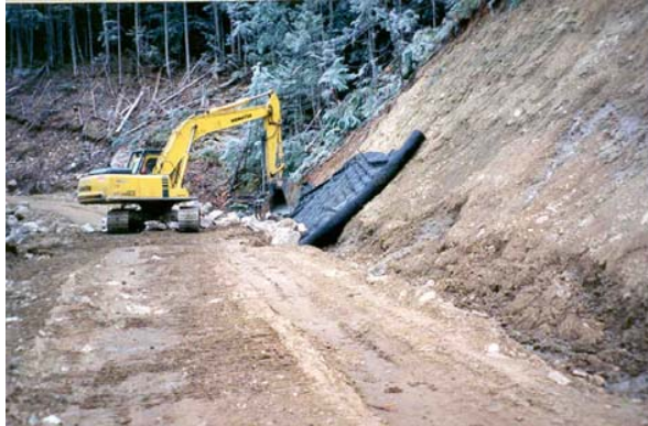
Figure 1. Geotextile installation over seepage horizon
