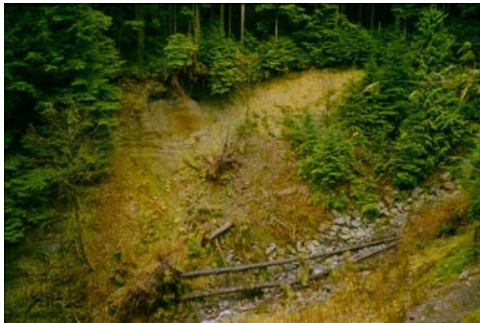
Figure 4. Incised channel with riprap stone (3 years after placement)
