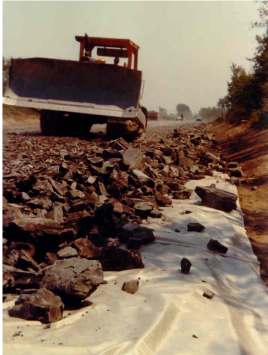
Figure-2: Photograph of attacked geotextile by aggressive cover soil
