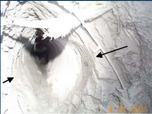
328-9 Abutment Stress Crushing/Stress Fracturing
