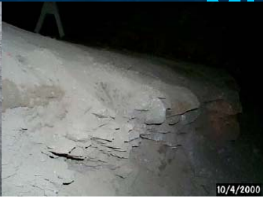
328-9 Abutment Stress Crushing/Stress Fracturing
