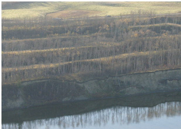
Figure 2. Aerial oblique showing multiple landslide blocks.
