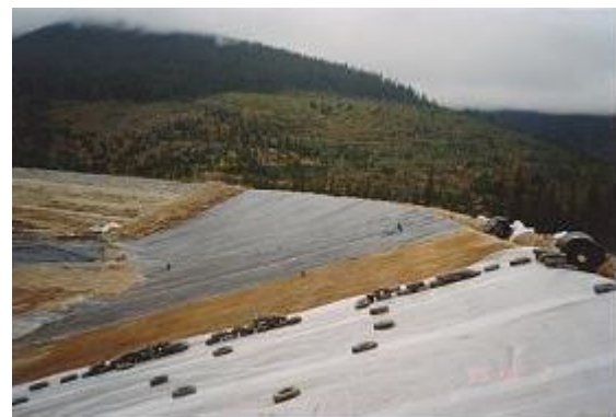
Figure 5: Coursier Dam – Installation of Geomembrane (1995)
