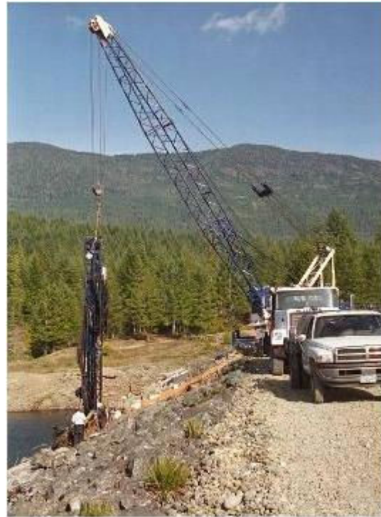
Figure 1: Crane-Assisted Becker Penetration Testing
