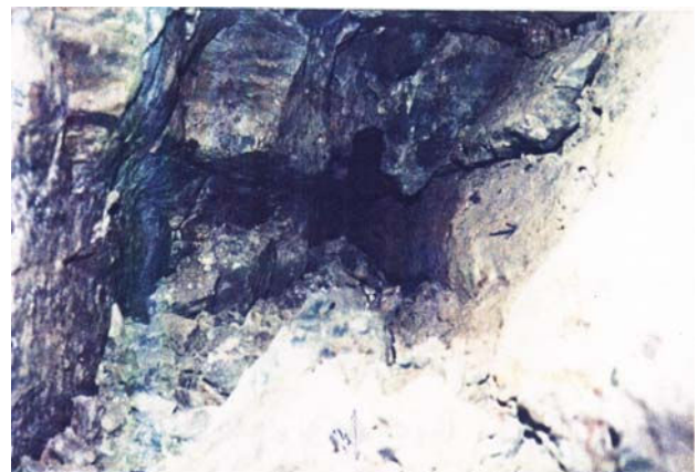
Figure 5. Boring a vertical shaft over the crest, C1 crossed the fault through the foundation
