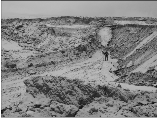
Figure 8a. Flank Failure (Crest)
