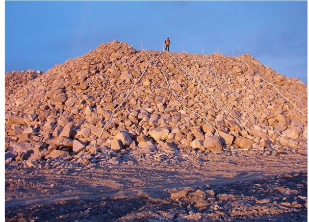
Figure 3. View on the front of test pile 2 during construction and placement of instruments in 2006 (Photo: Michael Gupton).
