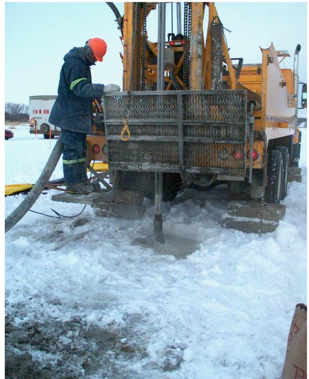
Figure 7: Drilling with air to start a borehole
