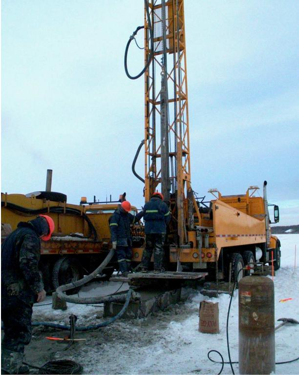
Figure 8: Installation of steel borehole casing
