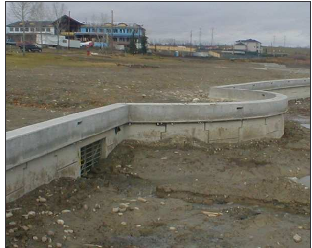
Figure 8. Chestermere Wall at Low Water (Note: Storm Water Drain through Wall)
