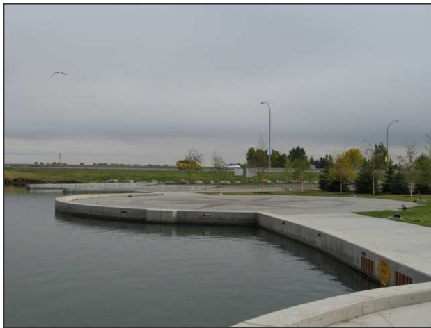
Figure 7. Chestermere Walkway at High Water (Note: Scupper Drains through Coping)
