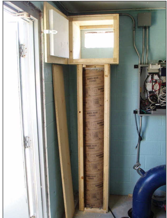
Figure 17. Total Station Enclosure Showing Concrete Support Column
