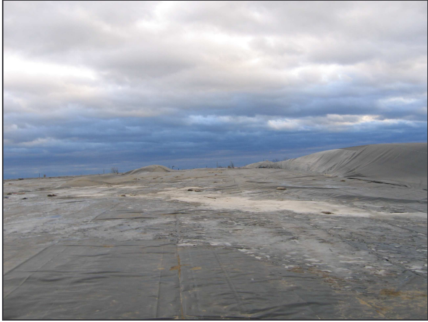
Figure 6 Photo of Wind Uplift on January 9, 2008
