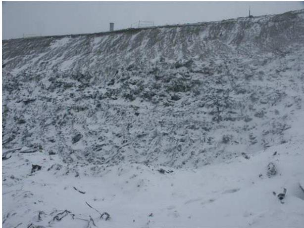
Figure 2. Slope steepened to 1H:1V
