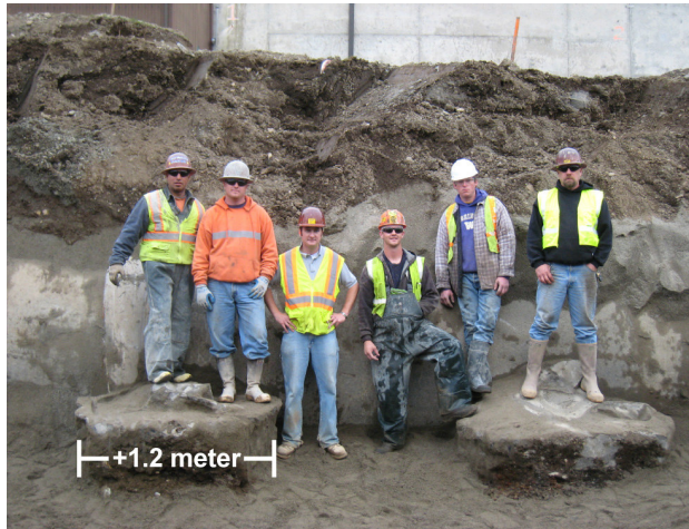
Figure 3. Exposed triple fluid jet grout column tops exceeding the design 1.2 m diameter
