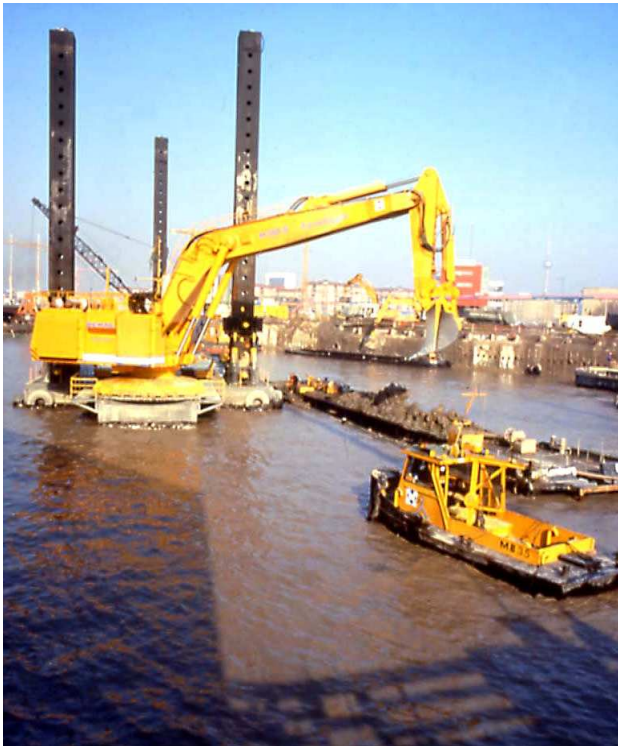
Figure 11. Excavation under water at Potsdamer Platz
