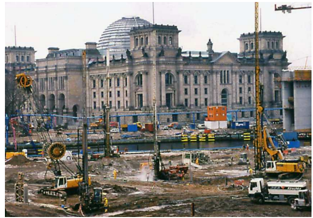
Figure 8. Deep excavation construction site with jet-grouted cut-off
