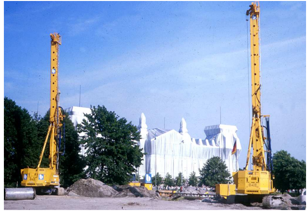
Figure 13. Removal of historic concrete structures with BAUER BG's by Bilfinger Berger AG
