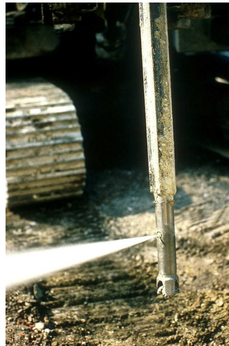
Figure 6. Soft gel grouting
