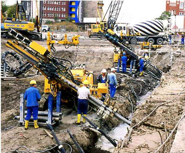
Figure 10. Ground anchor installation into diaphragm wall
