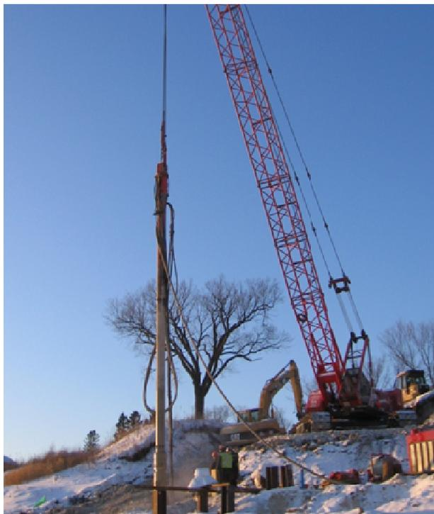
Figure 3. Compacting columns with vibrolance
