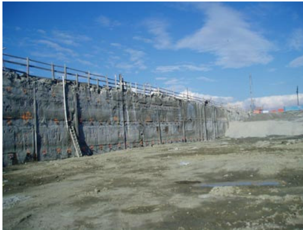
Photo 11- Excavated and trimmed jet-grouted wall
