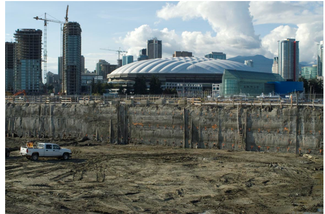
Photo 12- Excavated and trimmed jet-grouted wall
