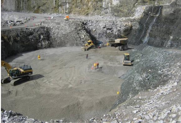
Figure 4. Spreading and roller compaction
