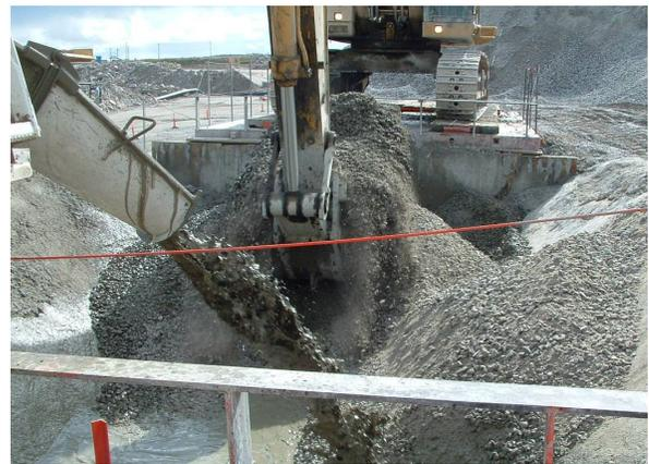
Figure 3. Pouring and mixing cement slurry
