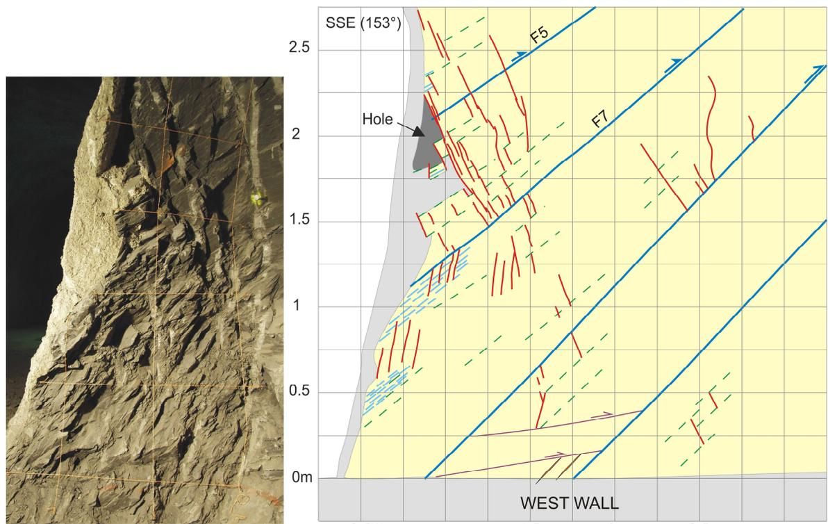
Figure 3. Induced fracturing in the east (top) and west (bottom) walls in the EZ-B Niche entrance (geological maps modified from Nussbaum et al., 2005a).
