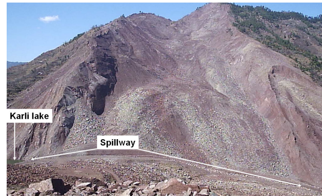
Figure 4. A pictorial view of open cut spillway at the landslide toe in front of Karli Lake (facing westwards)
