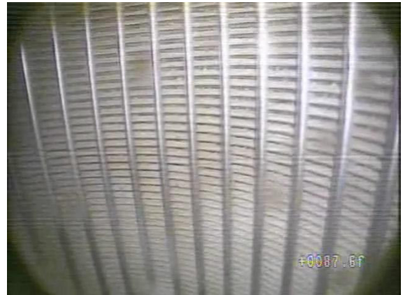
Figure 5B. 26.7 m looking sideways through the 30 slot screen. Medium sand grains are seen against the screen, forming a natural filter pack.
