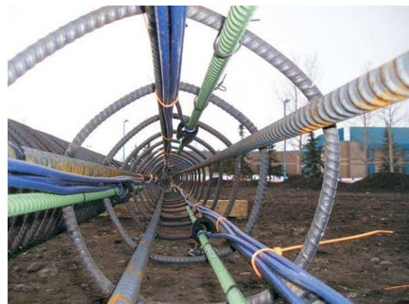
Figure 6. "Sister bars" installed on the rebar cage (note: leads bundled to vertical rebar)
