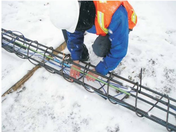
Figure 7. "Sister bars" offset from the vertical rebar
