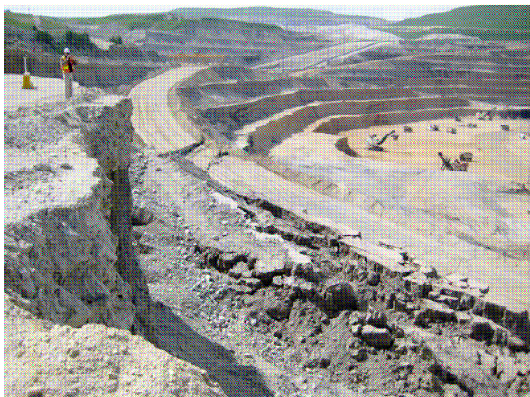
Figure 4. Looking down from the headscarp of the Lube Land failure (June 30, 2008). Note the high head scarp, smaller scarps across the haul road, and the wide 1115m bench occupied by the mining equipment.
