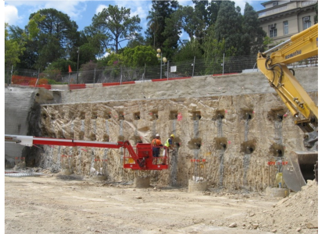
Figure 10. Installing dowels below Albert Street
